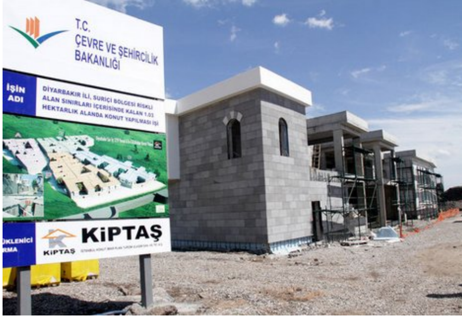
Photo 25: New houses being built in the old city Suriçi
