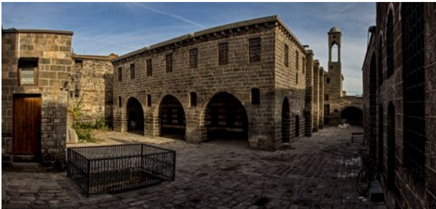
Photo 3: After the restoration in 2014
